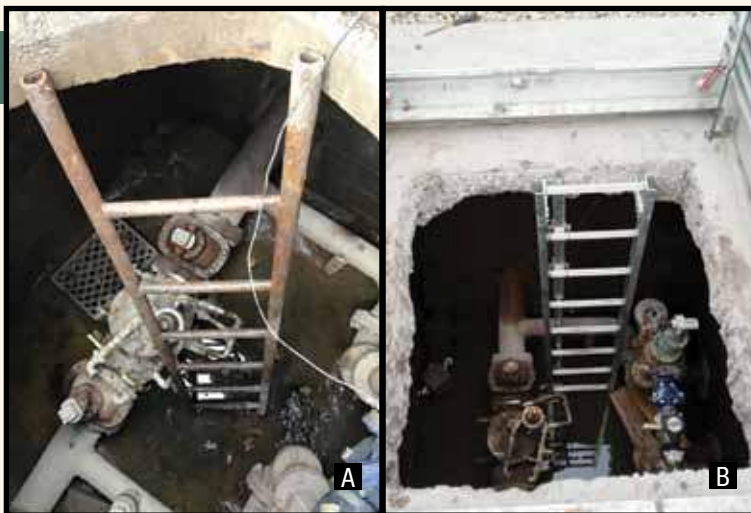
Local 648 Safety project: an example of a water regulation vault before (A) and after (B) with a new, secured ladder and entrance.
