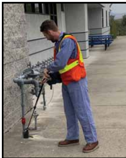
Chad Wadsworth, a Local 132 Construction Technician, performing a leak survey on gas distribution lines.
