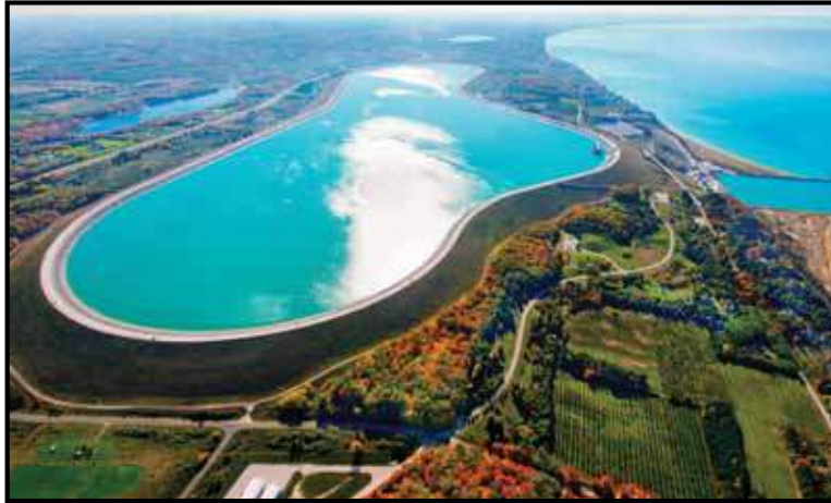
The Ludington Pumped Storage Plant sits on a 1,000-acre site along the Lake Michigan shoreline. The plant was built between 1969-73 and is jointly owned by Consumers Energy and Detroit Edison, and operated by Consumers Energy. Photo © Dale Fisher
