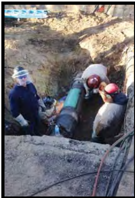
Local 483 members cutting and capping a 16-inch gas transmission line damaged by a third party contractor who was replacing telephone poles to restore services following disastrous mudslides.
