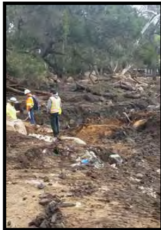
Montecito, CA suffered flash floods on Jan. 9 when torrential rains hit steep slopes denuded by a huge wildfire. Twenty-one people lost their lives and hundreds of homes were damaged or destroyed. A 22-inch gas transmission line buried 10 feet below the bottom of a creek was exposed by the flood and mudslide. Car-sized boulders like the ones pictured here tore it apart.
