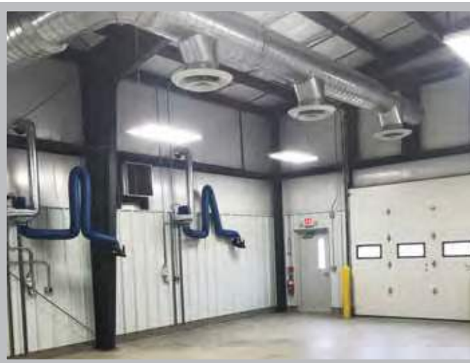
Building on this success, a new facility is being readied for opening to add welding training and more classroom space.
