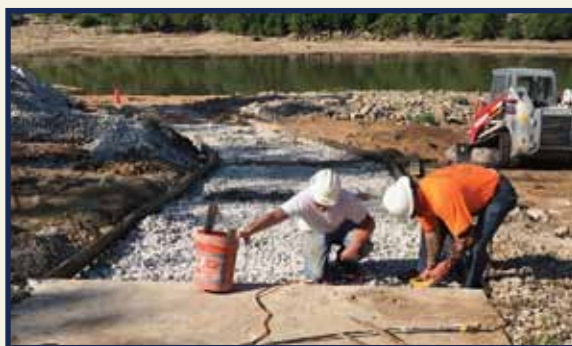
UWUA Local 335 volunteers from Missouri American Water, Nick Aulbach, left, and Dave Turner, reconstructed a boat ramp at Missouri's Minnie Ha Ha Park that was destroyed by flooding last spring.
