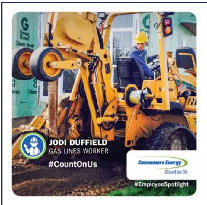
Jodi Duffield, a gas line worker and member of the Michigan State Utility Workers Council, shows her skills as part of a Consumers Energy ad.
