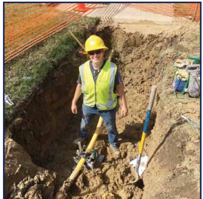
Kristen Baldwin, a gas line construction fuser and member of the Michigan State Utility Workers Council.
