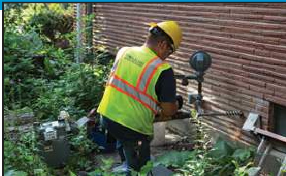
In Illinois, legislators approved funding for the Peoples Gas Accelerated Main Replacement Program in Chicago. Pictured here, installing new service for a residential customer.
