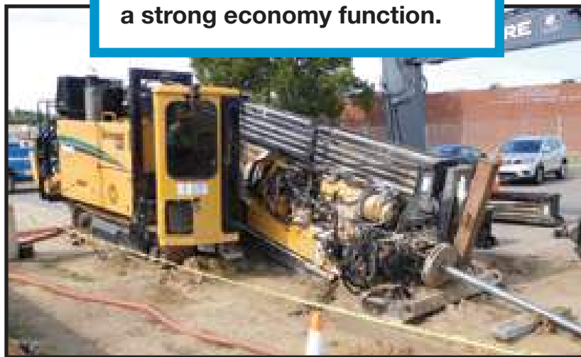
Michigan is investing in its gas infrastructure. Pictured here is a directional bore machine used to lay new gas lines as part of Consumers Energy's Enhanced Infrastructure Replacement Program.
