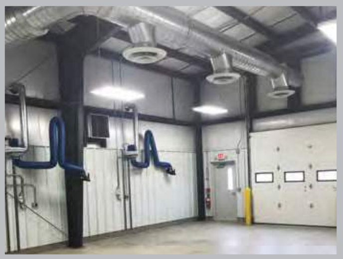
Building on this success, a new facility is being readied for opening to add welding training and more classroom space.
