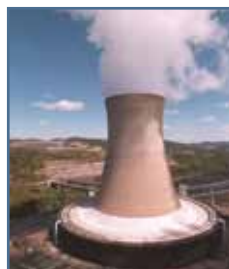
Harrison coal-fired power station, WV. (AP Photos)
